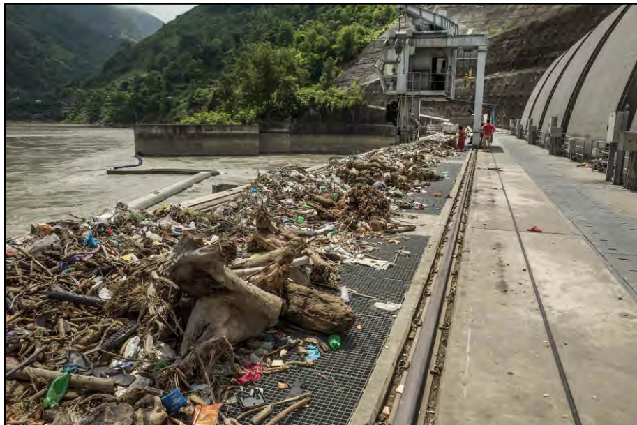
Figure 20: Photograph of debris removed from trash rack on Kali Gandaki hydropower plant in Nepal.
