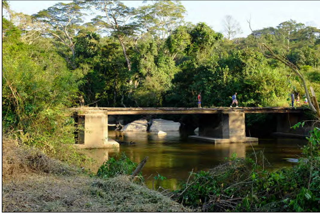
Figure 6: Kolba City bridge streamgage location (photo provided by LHS).
