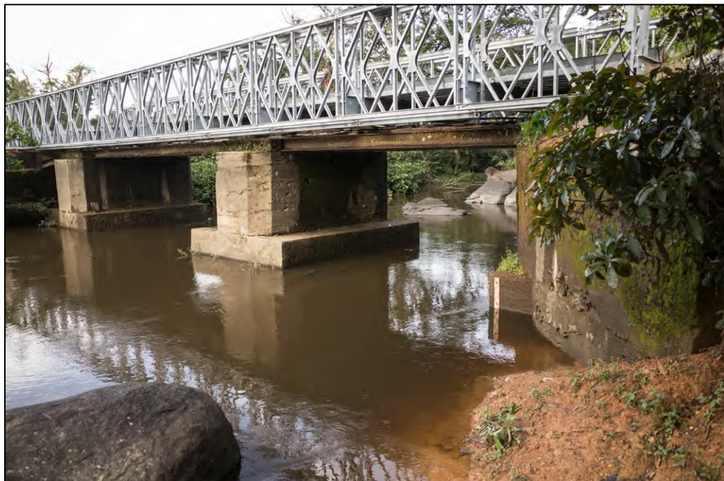
Figure 5: Kolahun bridge gage site, looking upstream, staff gage visible on the abutment on the right side of the photo (downstream side of the bridge).
